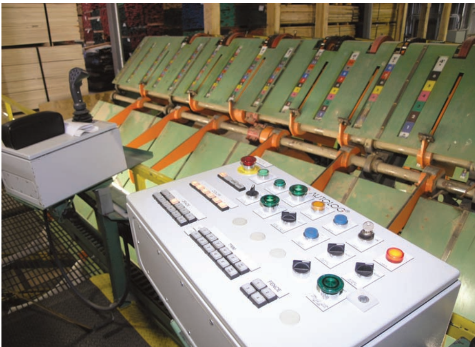
The TS Manufacturing grading stations are placed to give operators a great view of each piece. The flow is split between two grading lines, each with surge deck.
